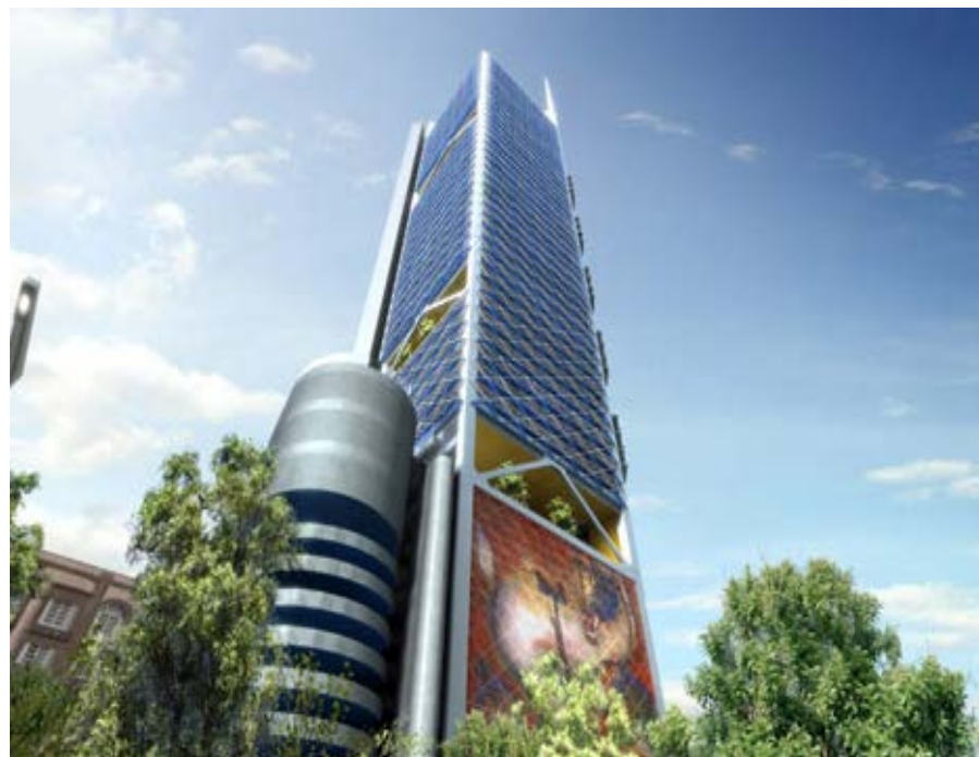
Future BBVA Bancomer Tower under construction in Mexico City.
